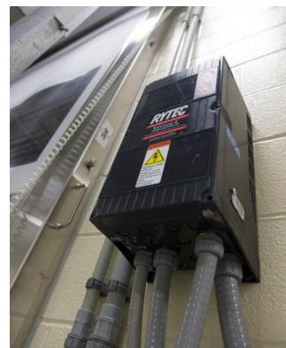
▲ System 4 controller. AGV control system communicates with door controller.
