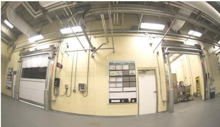
▲ Positive Pressure. The air flows from packaging to the warehouse to shipping and out the loading dock doors.
