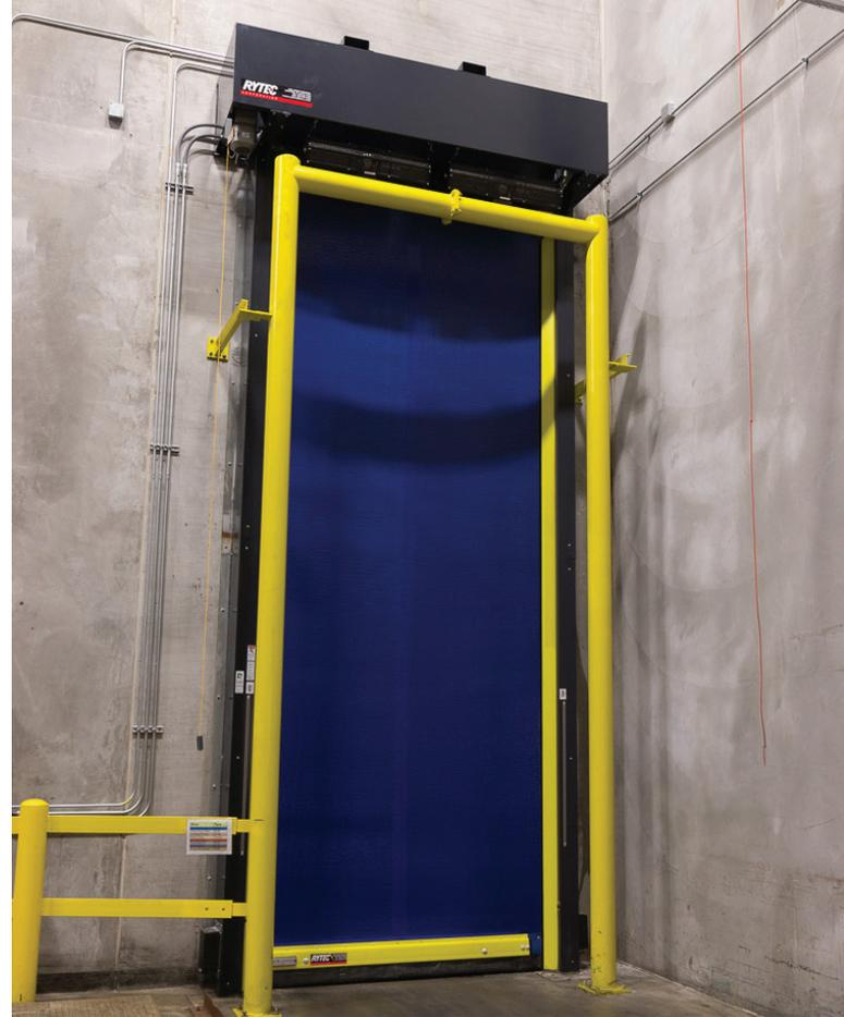
The older roll up doors at Palermo's have solid bottom bars. The soft bottom bar on the Rytec Turbo-Seal doors conforms to the contours of the plant floor, providing a much more effective energy-loss barrier.
