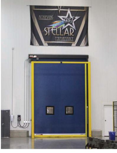
The Rytec Ry-Wi™ system is an example of this advanced thinking. This idea eliminates the coil cords usually attached to the bottom bar and communicates continually with the System 4 controller – wherever the controller is mounted – to continually track door operation and provide greater safety.
